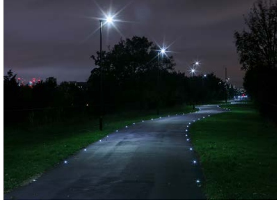
Newham Greenway - edge installation
